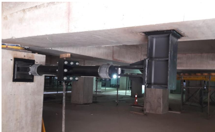
Fig 10: Final on-site assembly of the coupled FVDs
